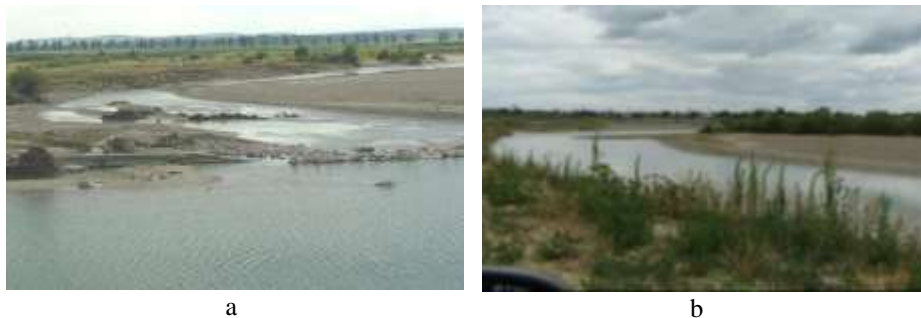
Fig. 7 – Current status of the secondary riverbed: a - the input sector; b - the central sector.
