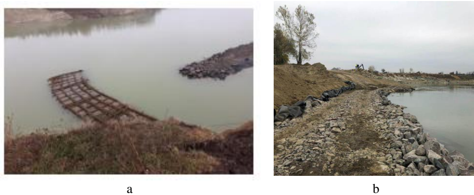
Fig. 6 – Overview of the Siret River, Slobozia Galați County, year 2018: a - lifting the fascine mattress on the Siret River, Șendreni commune; b - shore consolidation of anchorages on the Siret River, Șerbești commune (A.B.A. Prut–Bârlad, 2018).
